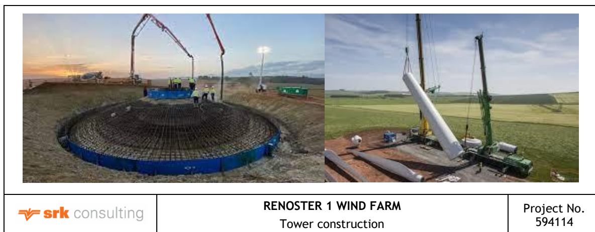
Figure 2-17: Construction of a crane pad foundation (left) and tower sections being craned into position (right)
