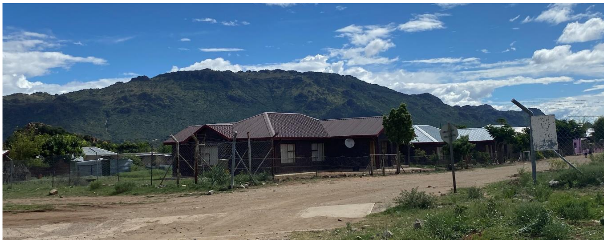
Figure 4-3: Brakfontein resettlement houses
