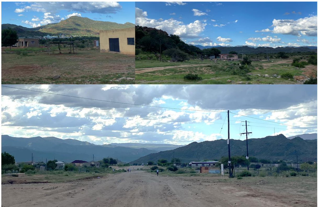
Figure 4-11: Dwellings in the mine's Aol
