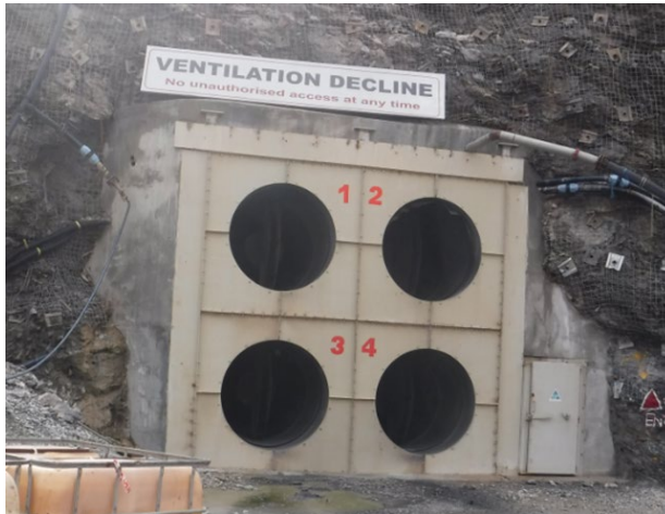
Phase 1 fan installation 4 x CC1400 fans
