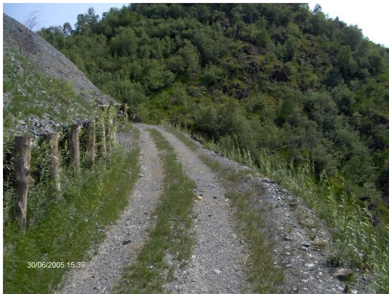
Fig. 5: Planted and seeded « pathway » after completion.
