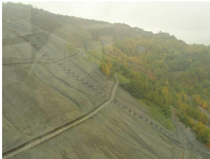
Fig.7: Aerial view of the site. Horizontal pathways and one water chute are visible, as well as pre-existing deep erosion features.
