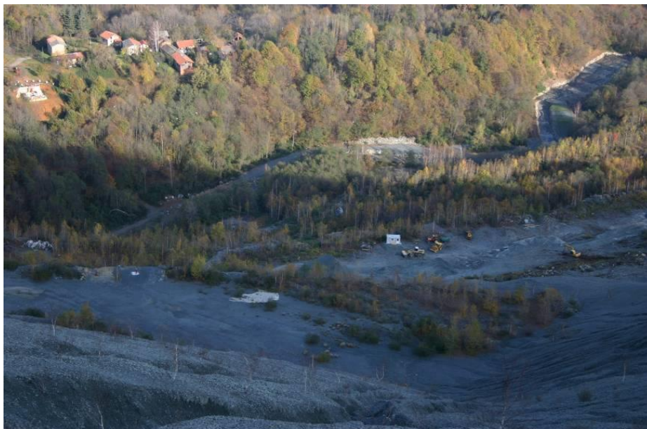
Fig. 2: Looking down slope: nearby houses, the Fandaglia Creek and the decant basin
