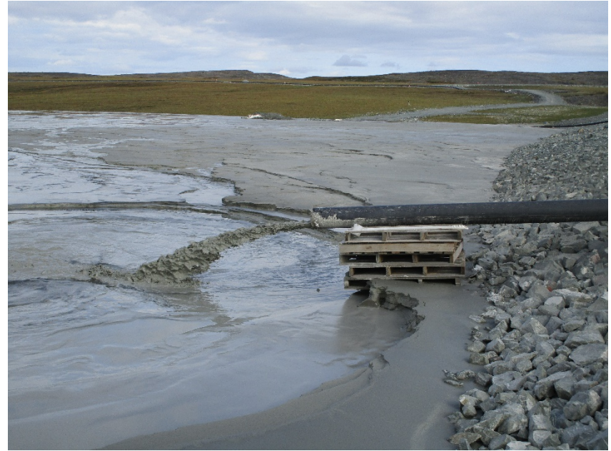
Tailings discharge from spigot along upstream face of dam
