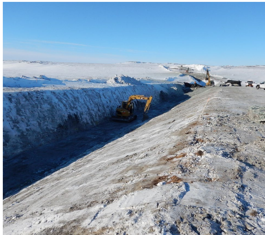
Near complete section of key trench
