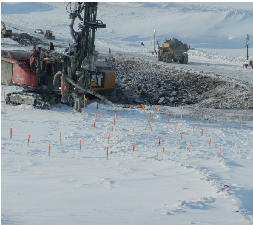
Foreground: Drilling of blast holes Background: Key trench excavation
