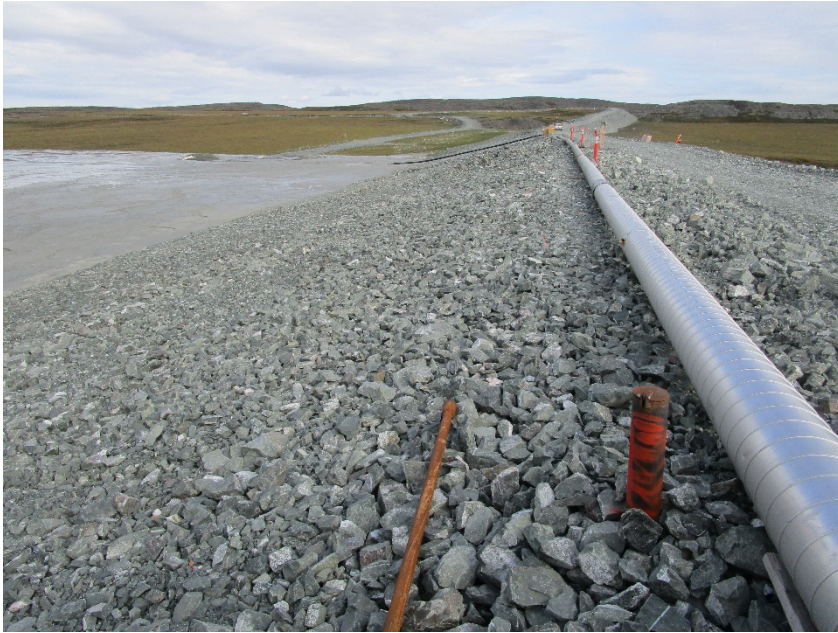
Tailings discharge line along crest of dam
