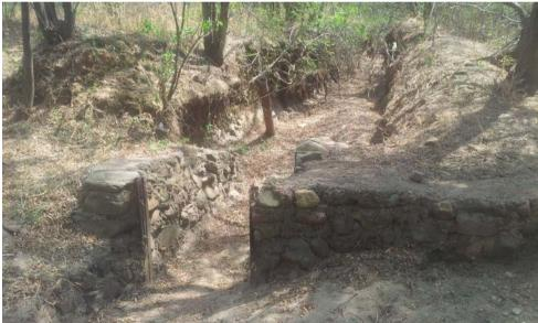
Figure 31: Start of the canal (furrow) off the Magalies River with sluice opening clearly visible
