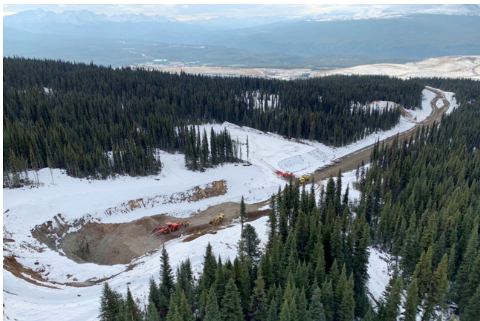
Figure 5 Access Tunnel South Portal Location (October, 2018)
