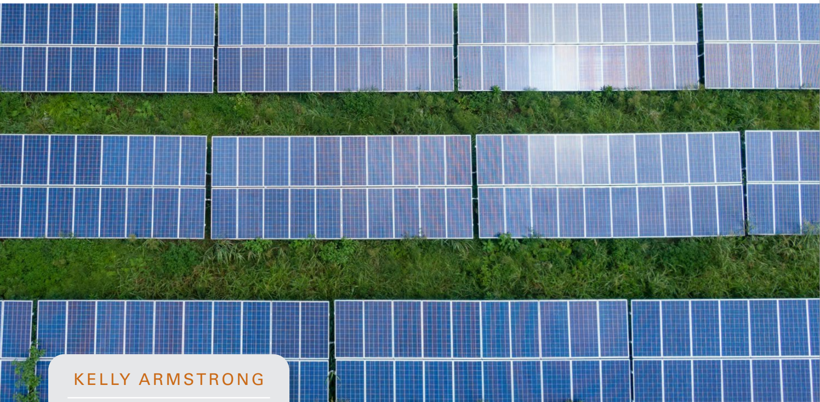
Light reflecting (glare) off PV panels.
