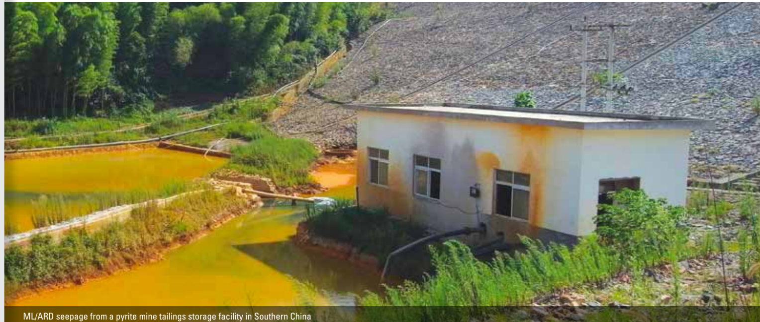
ML/ARD seepage from a pyrite mine tailings storage facility in Southern China
