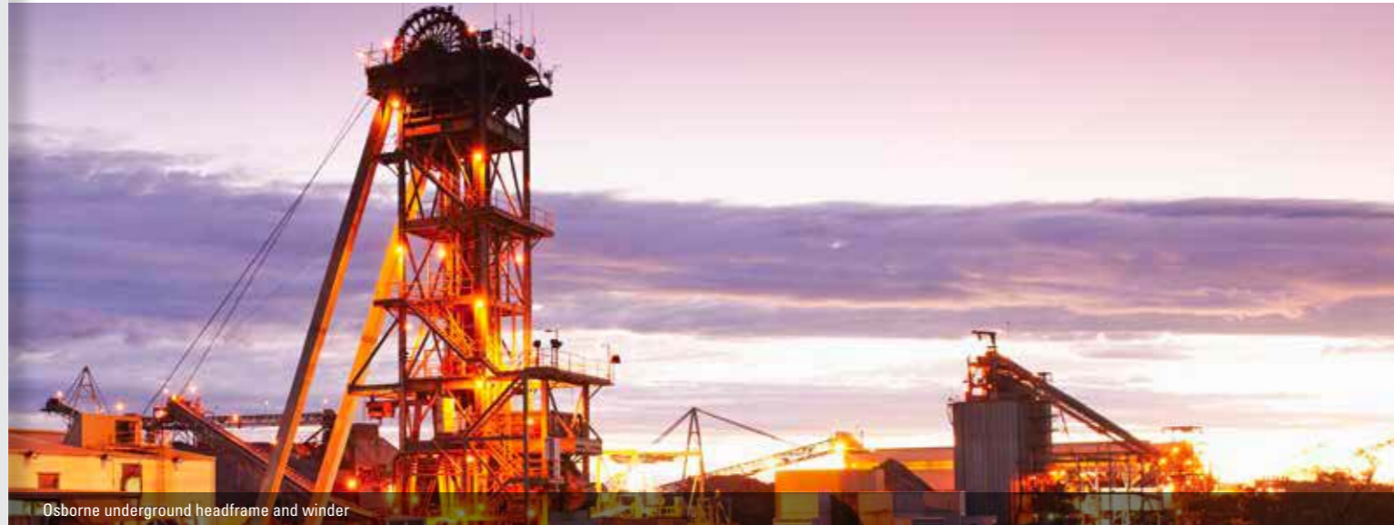
Osborne underground headframe and winder
