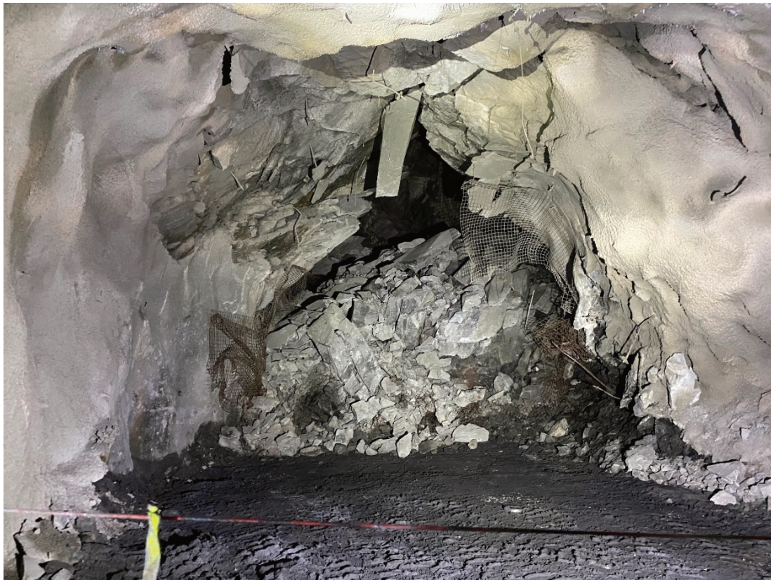
Figure 2 Level 1079 footwall drift looking north showing fragmentation from the back and a void above the rock pile
